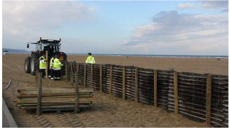
The construction of wooden fencing topped with dried heather along the beach walkway of Deauville to limit blown sand and thus limit walkway maintenance.
