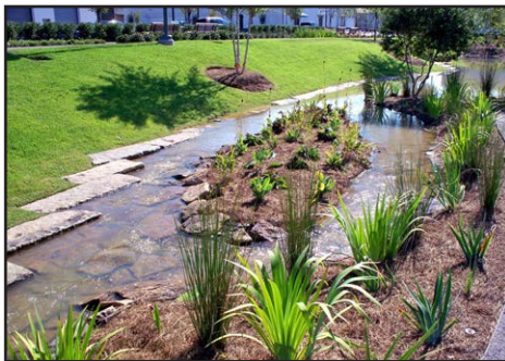
Stormwater Drainage Gardens
