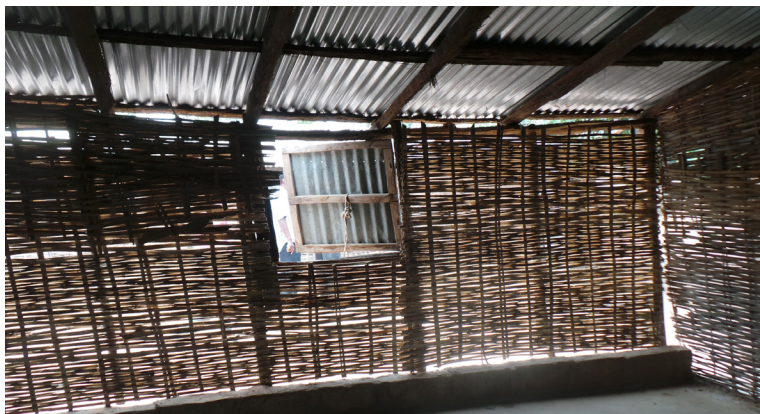
Interior of a classroom. Walls made of woven bamboo, zinc for the roof, and a metal panel to close the window.
