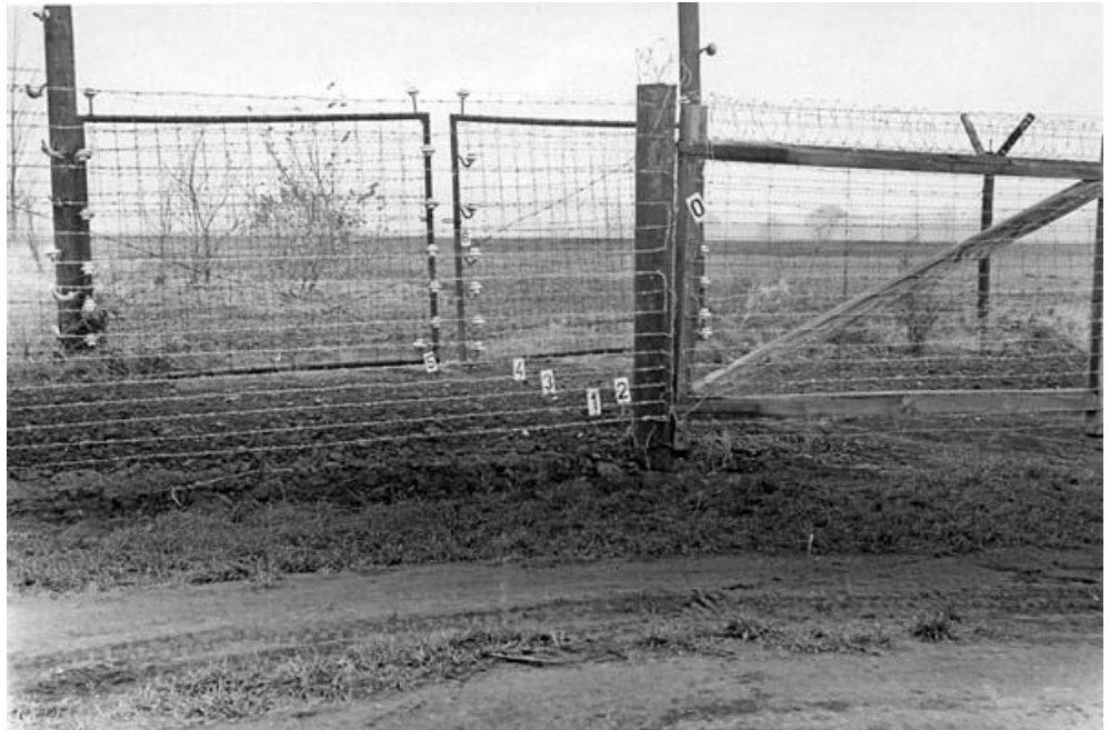
Internal borders of the restricted zone. No sign pointed to the electric fence
